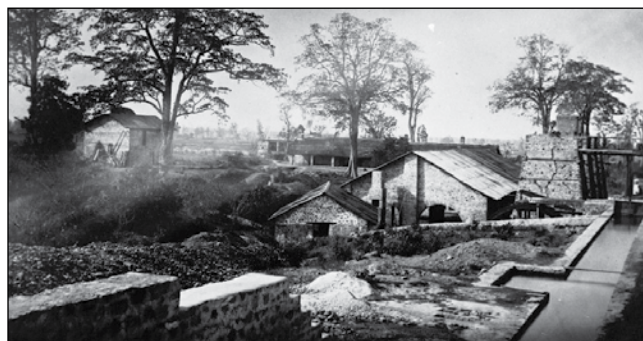
Kumaon Ironworks at Kaladhungi
