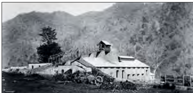
Blast Furnace at Dechauri (1862): height approximately 10.2 metres (34 feet) by William Sowerby, in working condition when Julius Ramsay arrived in 1861. In this furnace, approximately 400 tons were made in 1862-3 under Ramsay's supervision
